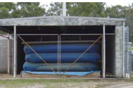
Biogas collector at Foster's Australia.
