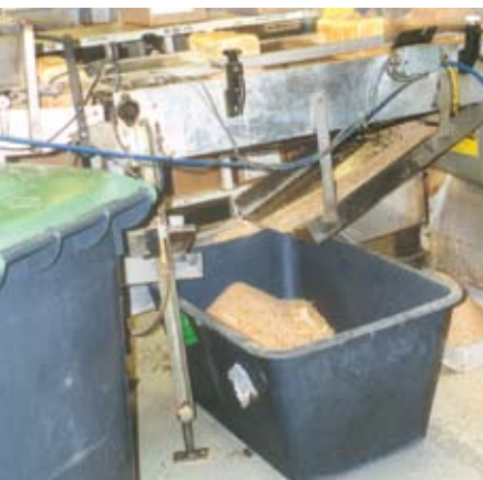
Collection of bread crumbs for reuse in the process
