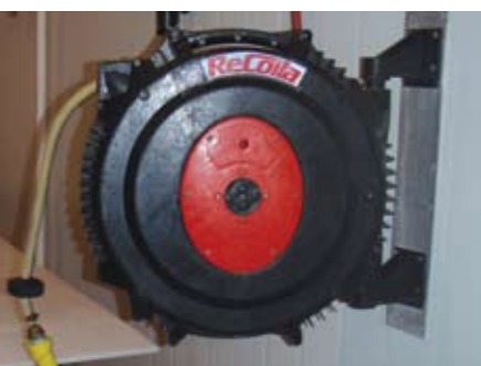
Automatic reel-up hoses reduce accidental damage to hoses.
